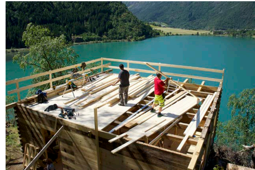
Views down the Fjord and laying the floor
