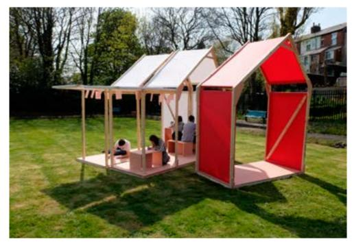
Group 12 - Palletable Playground: The pavilion has been designed as part of a pilot scheme, transforming the Smith's Rec site from a troubled area to a rejuvenated space, safe for children and families. Designed in panels to be easily deconstructed and reconstructed.
